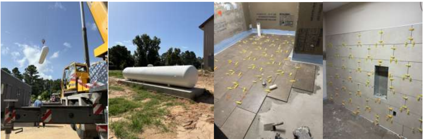
Propane tank delivery and set-up
