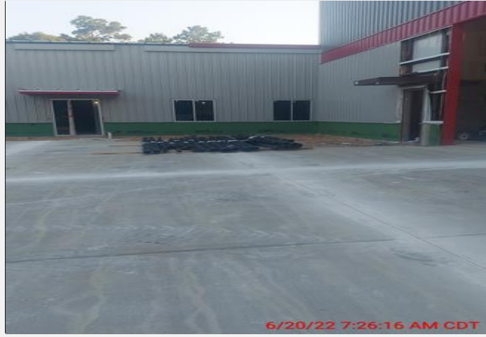
Fire Sprinkler Piping
