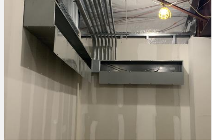
Electrical Gutter Boxes
